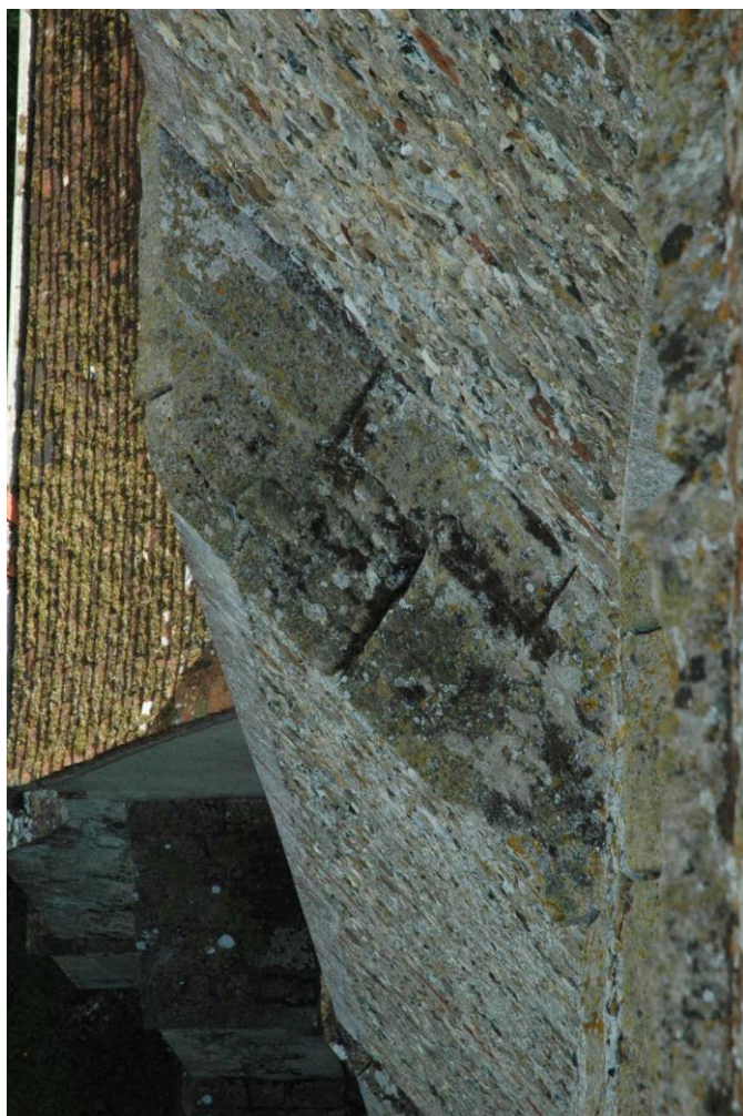
Pointing open joints to the tower when the cost of access is justified. Chute board rotting.
