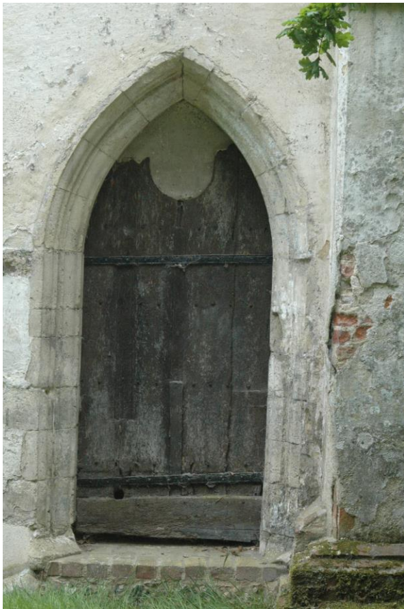
The old flue outlet!
