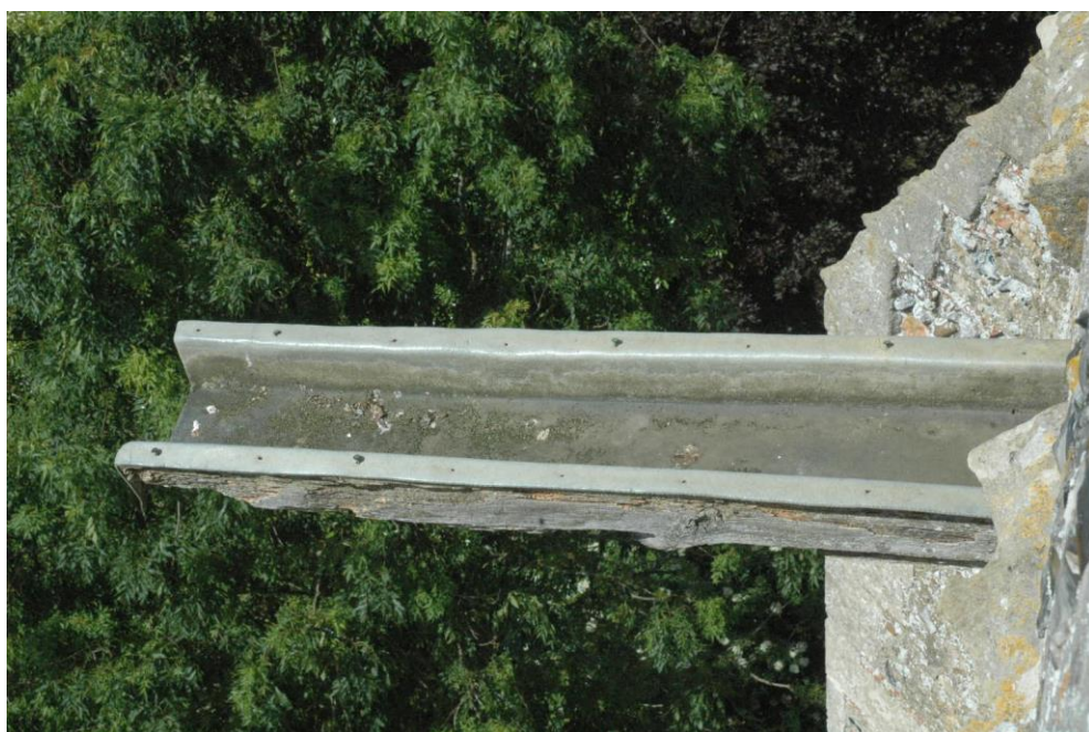
Pointing open joints to the tower when the cost of access is justified. Chute board rotting.
