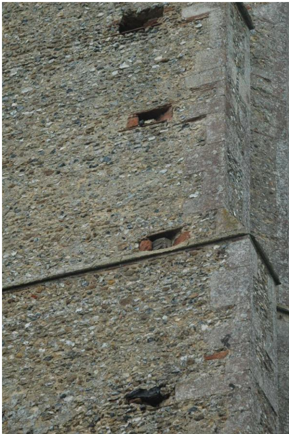
Block putlog holes from inside.
